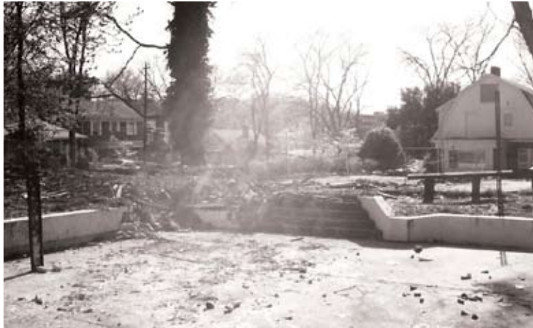
This photograph was taken in early summer of 1993. The White House had been torn down and construction of the new social quarters was about to begin.
